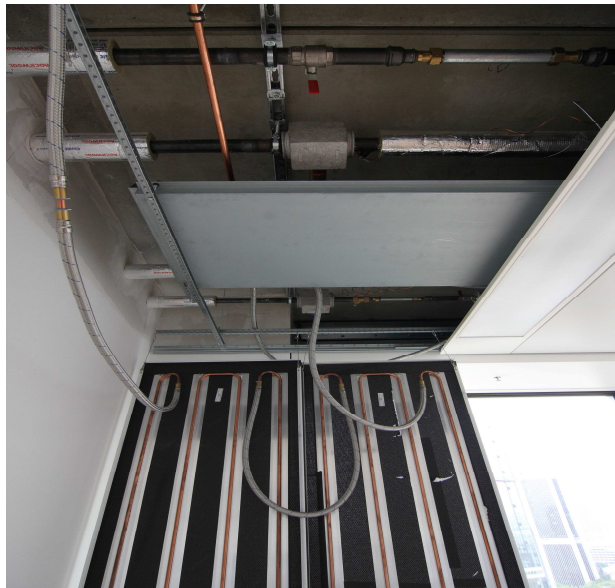
Hybrid ducts above the Ceiling panels, lowered panel
