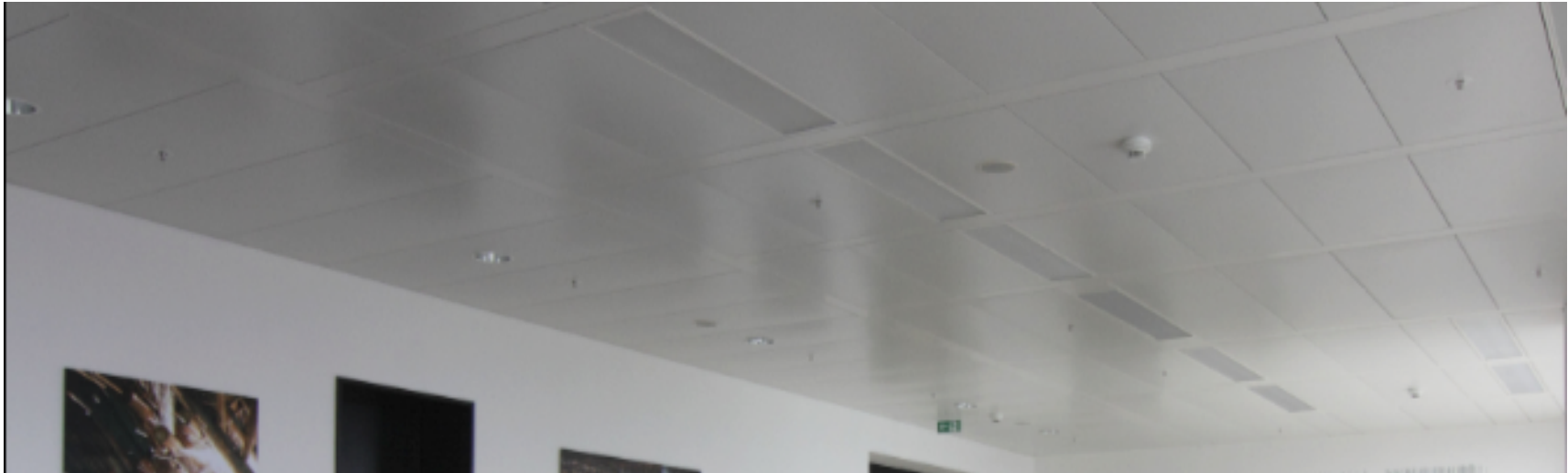
Hybrid Cooling Ceiling A11 Hybrid with Tape Grid Model
