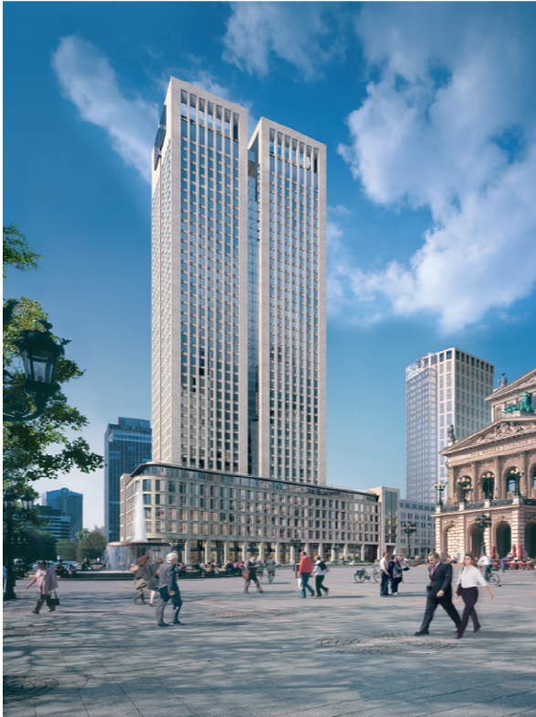
Opernturm, Frankfurt 41'000m 2 activated surface
