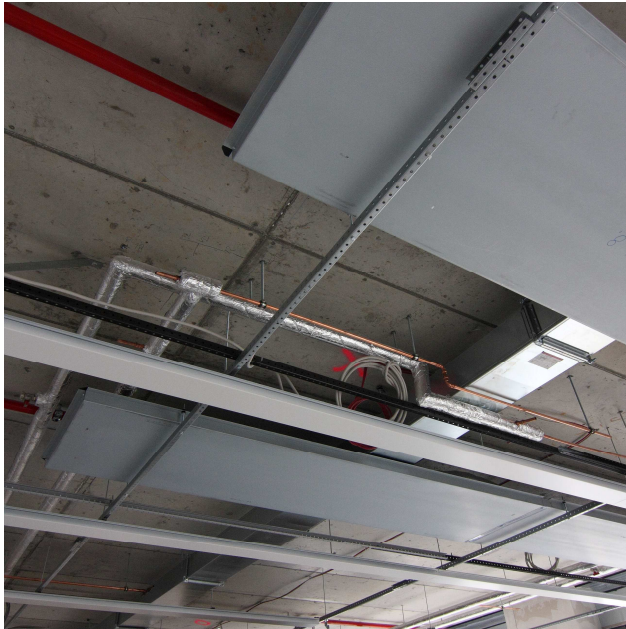
Hybrid ducts in ceiling cavity Arranged to window
