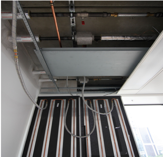
Hybrid ducts in the ceiling cavity, cooling plates swung out
