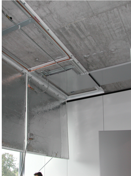
Hybrid Module U45 Hybrid Cooling plates swung out
