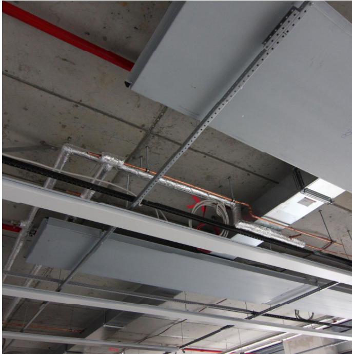
Hybrid ducts in the ceiling cavity aligned to the window axis
