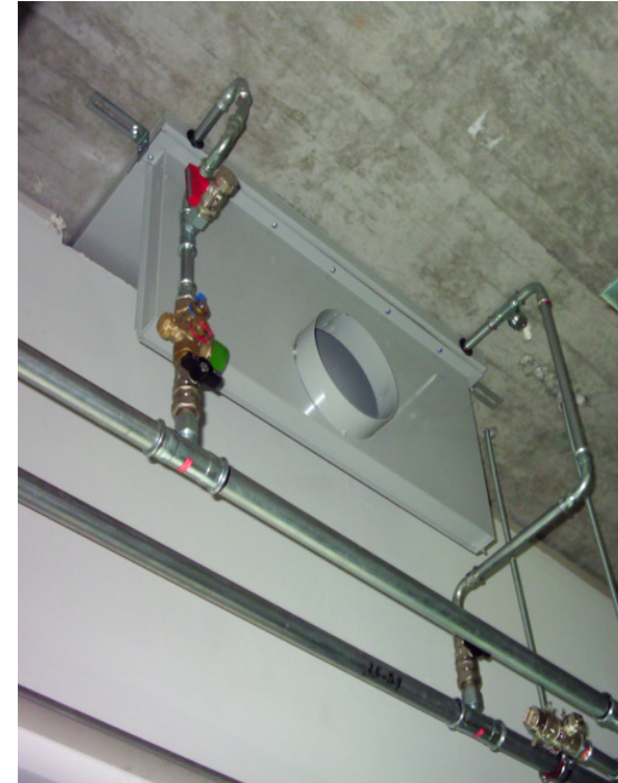
Ventilation connection section in the ceiling cavity (floor)
