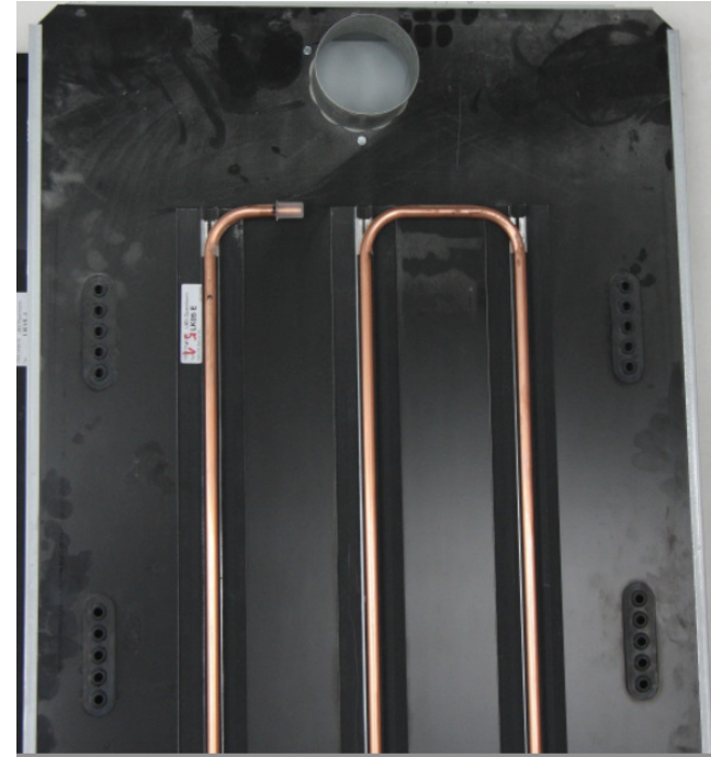
Hybrid ducts, view from above, Activation – air pen stocks
